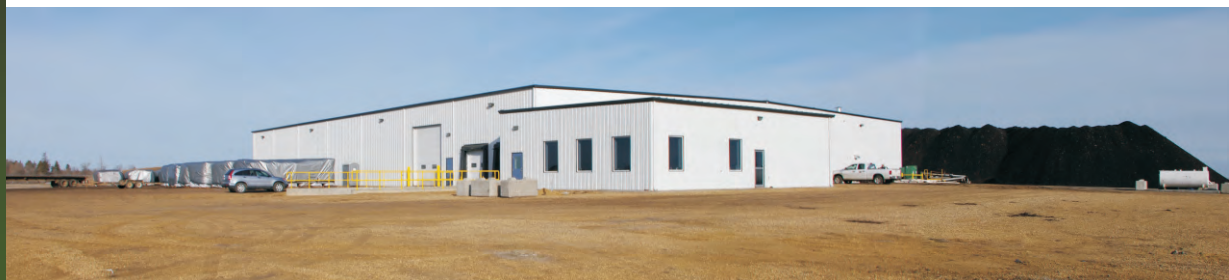
Black Earth Humic Production Facility in Ryley Alberta, Canada
